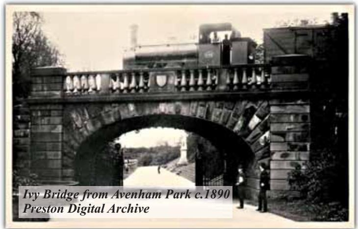
Because of the limited height it has an elliptical arch and crosses the Broad Walk between Avenham and Miller Parks on a 30 ft. skew over to the south-west, 12 ft. from the square. The parapets comprise bulbous cast iron balusters with stone copings, and alternate stone panels; there being four sets of four balusters on each parapet, with a half baluster at the end of each stone panel and parapet end.
